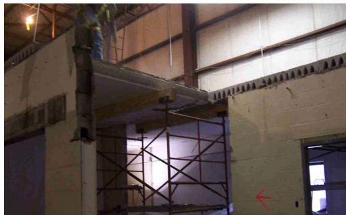
Walls coming down
