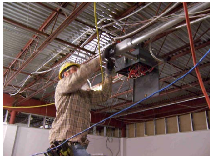
Lots of wires to move - telephone, internet, alarm system
